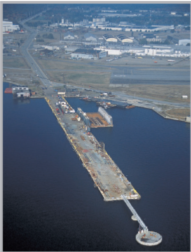
Senesco's docking and dry dock facility at Quonset Point Industrial Park.
