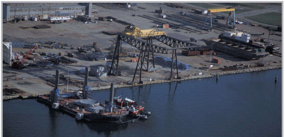
Transporter yard where barges are rolled into the water.
